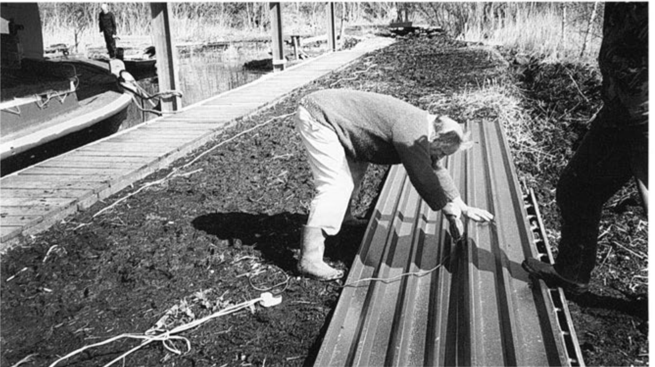
Cladding for the wet boatshed being prepared ready for installation
