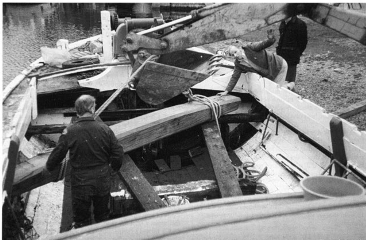
Main beam being lowered into place on Albion
