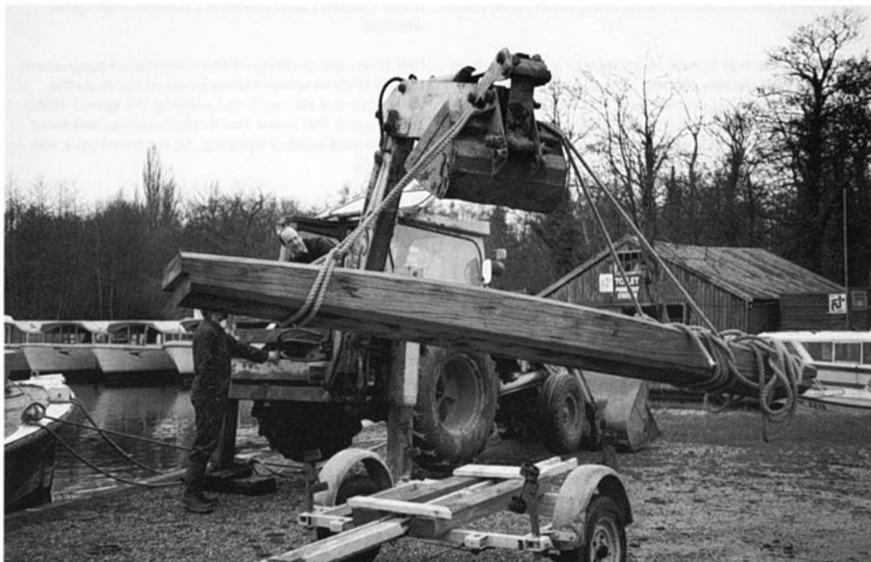
The new main beam being raised from its trolley. 1985-1986
