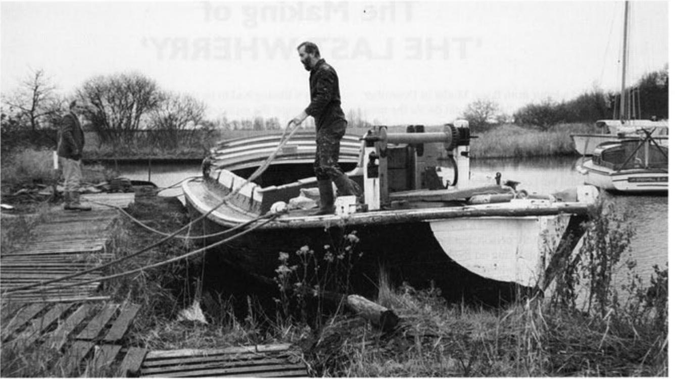
The wherry base before pathways, quay heading and wet boat shed had been installed. Notice the duckboards to keep your feet above water!
